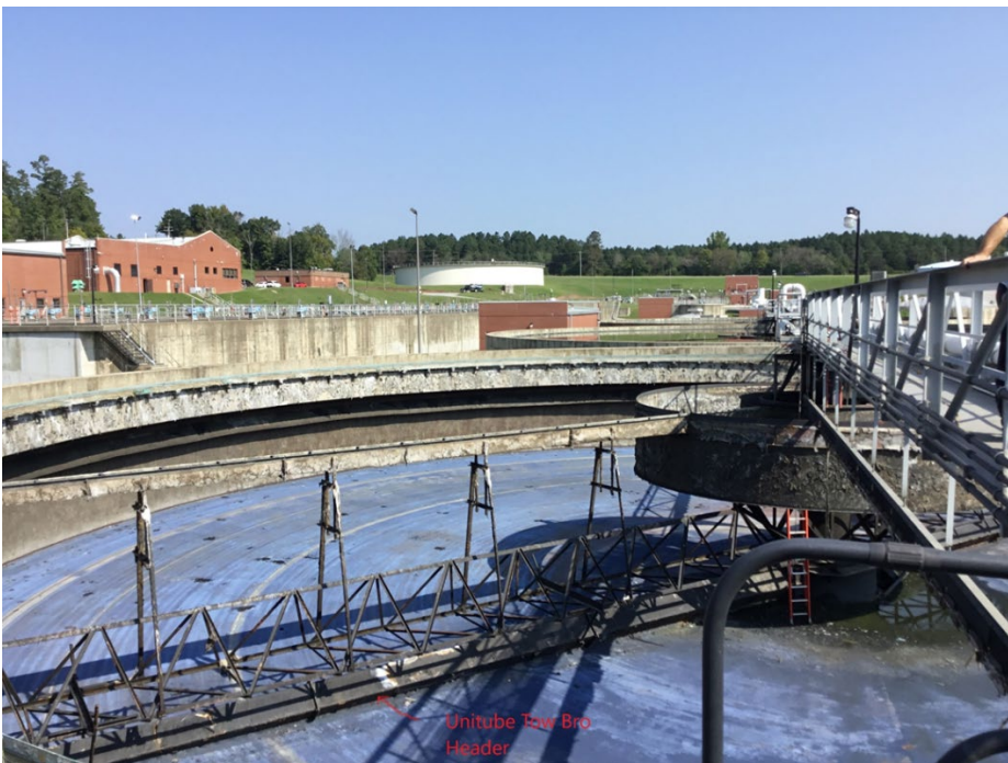
View of a drained final clarifier
