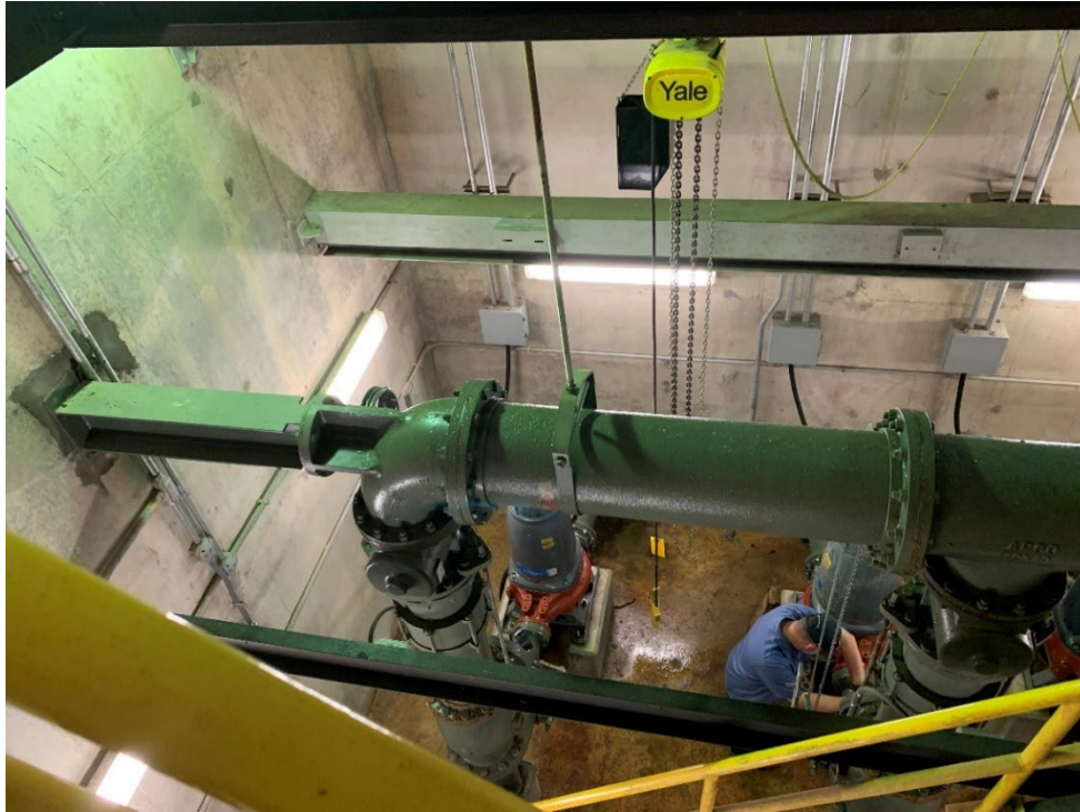
Dry Well of the Shadybrook Lift Station
