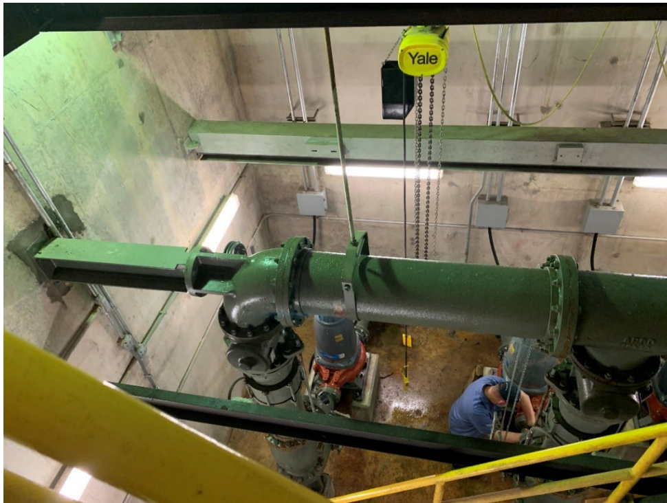
Dry Well of the Shadybrook Lift Station
