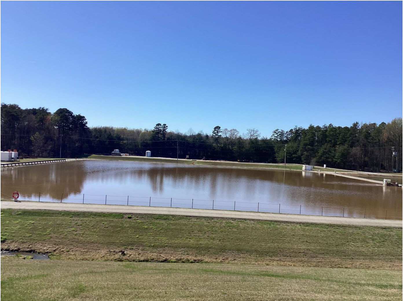
South Lagoon at the Ward Water Treatment Plant
