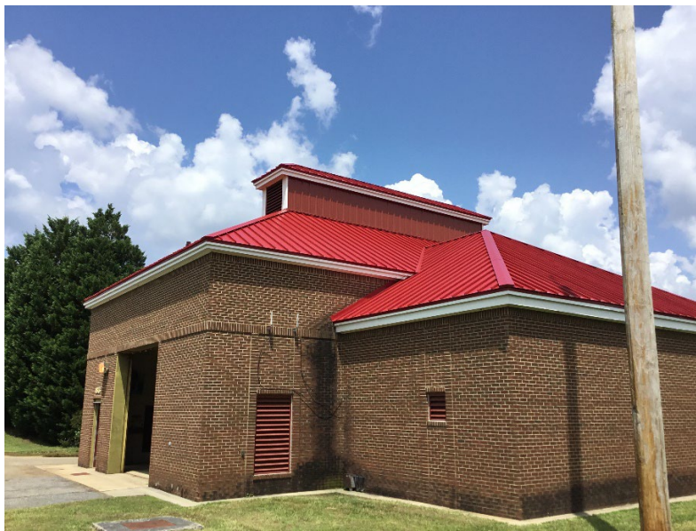
Oak Hollow Raw Water Pump Station
