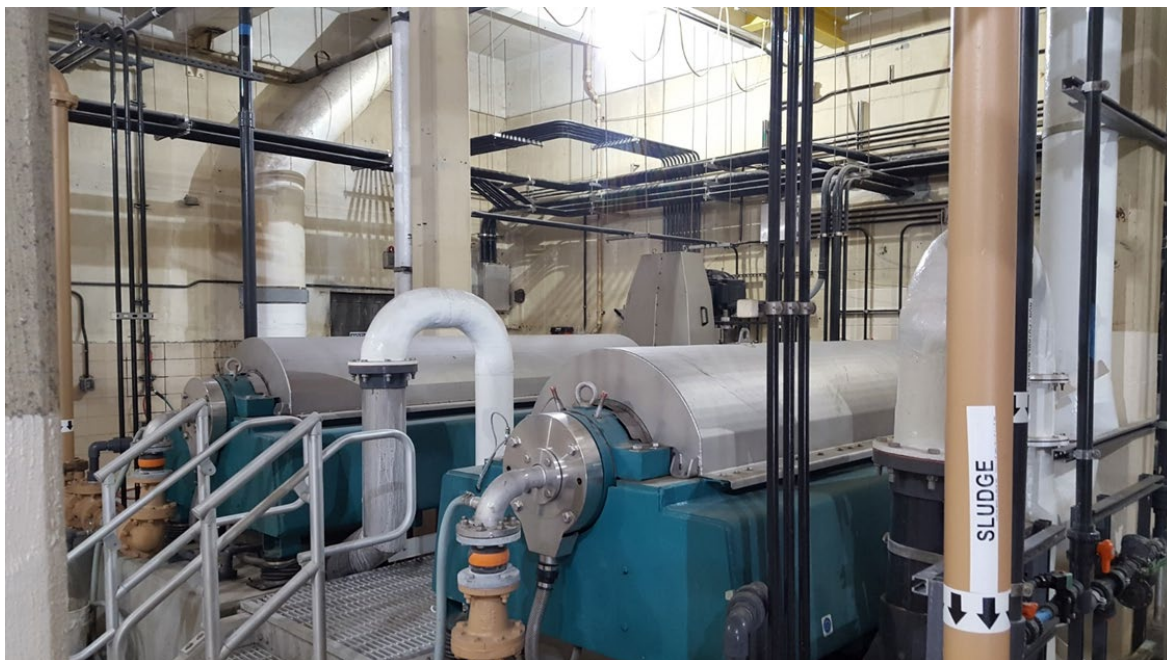
Centrifuges 1 and 2 at the Eastside WWTP
