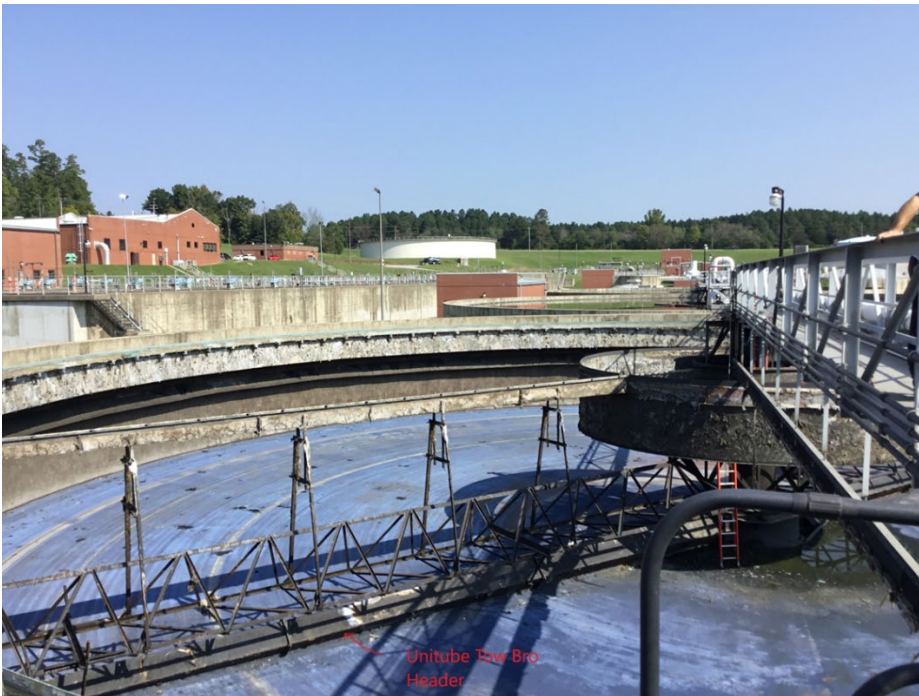
View of a drained final clarifier
