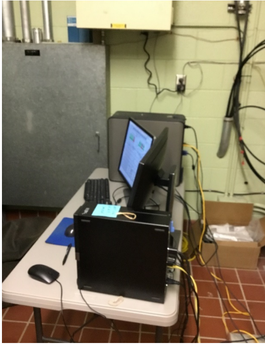
Outdated SCADA computers and communication connections
