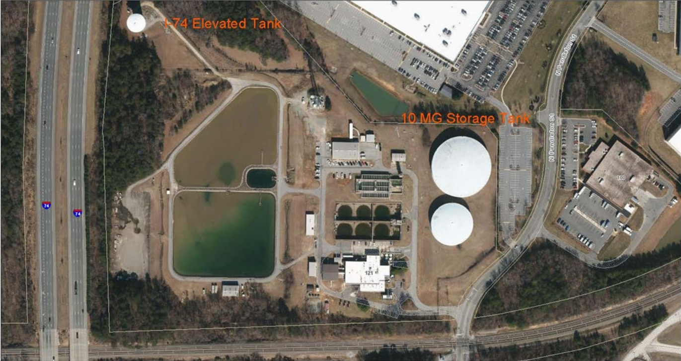
Aerial View of the Ward Water Treatment Plant
