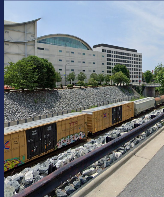
NCRR SLOPE STABILIZATION ALONG BROAD ST.
