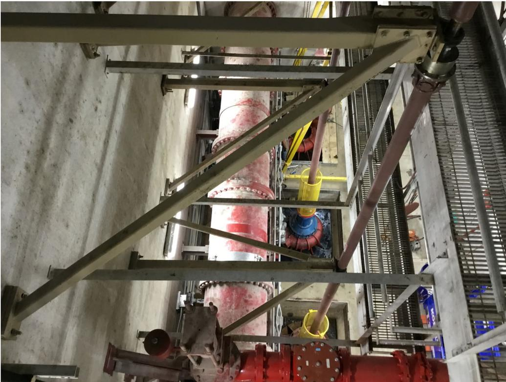
Picture of the 3 screw centrifugal pumps and drive shafts in the Riverdale Pump Station dry well.
