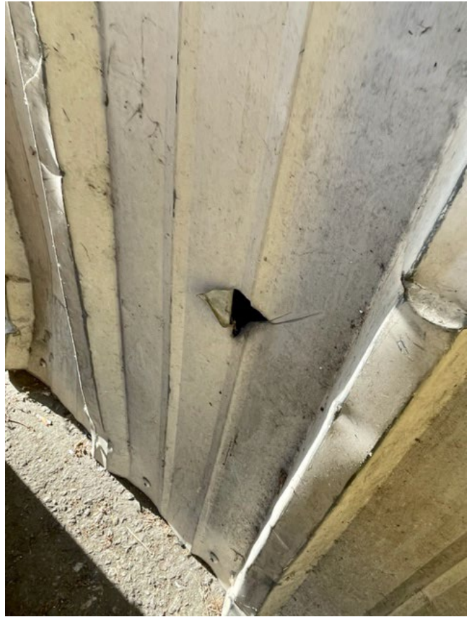
Pictures of damaged exterior siding
