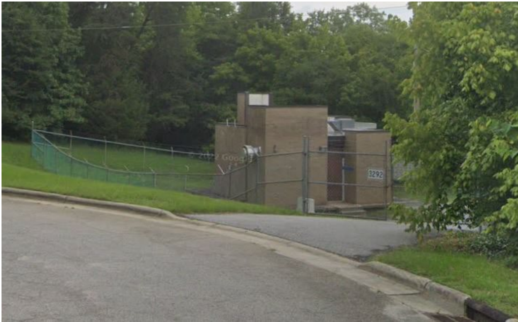
Shadybrook Lift Station
