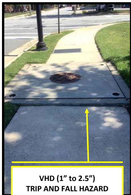
VHD (1" to 2.5") TRIP AND FALL HAZARD Repairable using Precision Concrete Cutting Process
