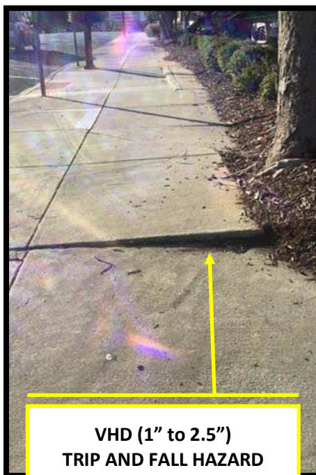
VHD (1" to 2.5") TRIP AND FALL HAZARD Repairable using Precision Concrete Cutting Process
