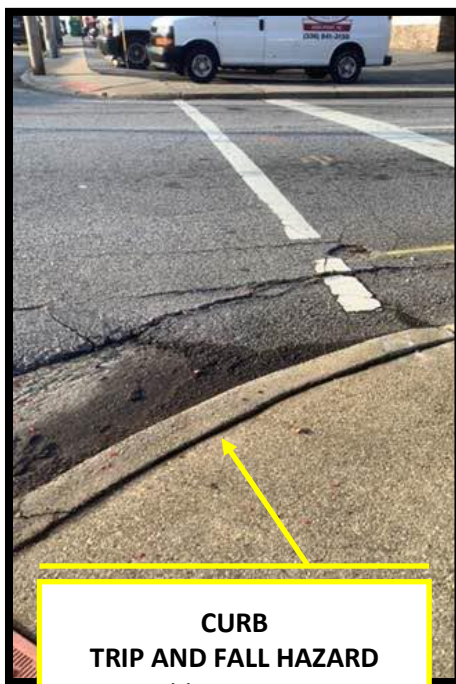
CURB TRIP AND FALL HAZARD Repairable using Precision Concrete Cutting Process
