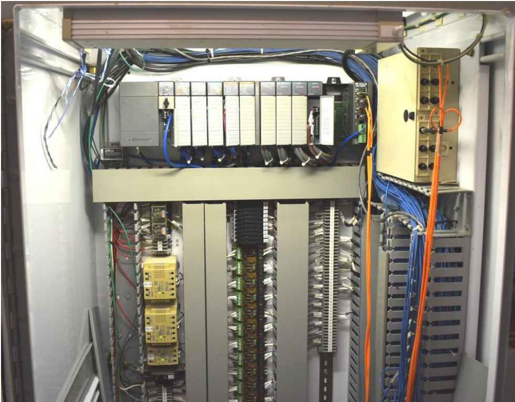
Example of a PLC cabinet that will be replaced as part of the project.
