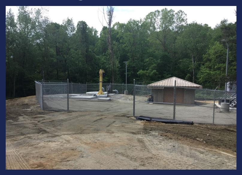
Construction of a new lift station with a peak capacity of 4.2 MGD and approximately 16,577 LF of 18-inch force main.
