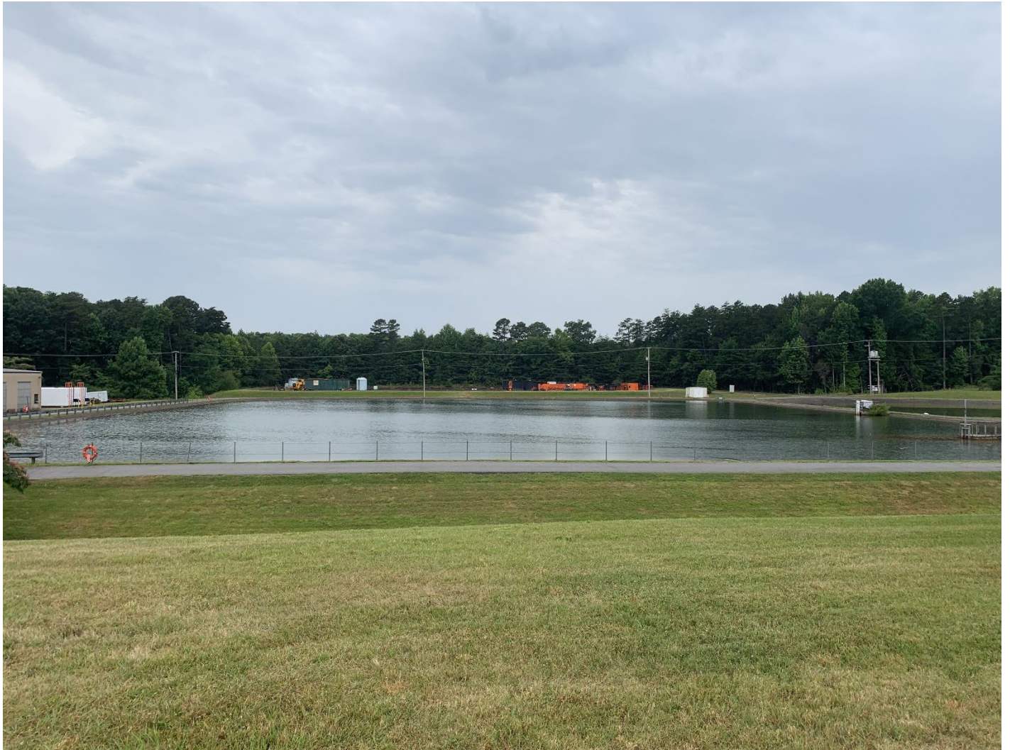
The south lagoon at the Ward Water Treatment Plant upon completion of the dewatering project.
