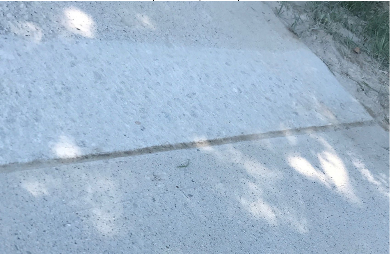
Trip Hazard Repair Example
