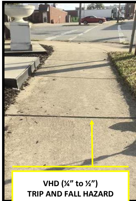
VHD (¼" to ½") TRIP AND FALL HAZARD Repairable using Precision Concrete Cutting Process
