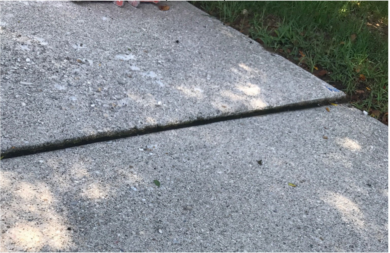
Trip Hazard Repair Example
