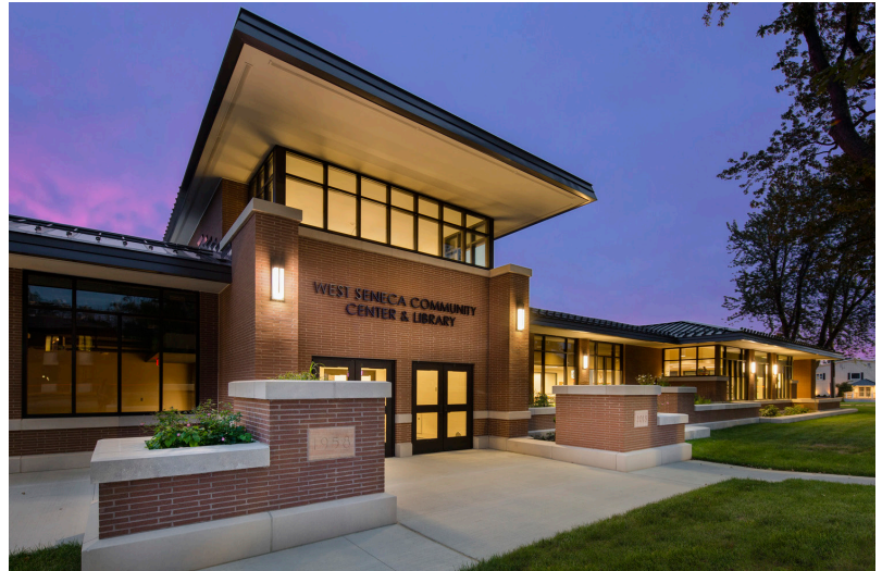
Town of West Seneca Community Center and Library Expansion, West Seneca, NY
