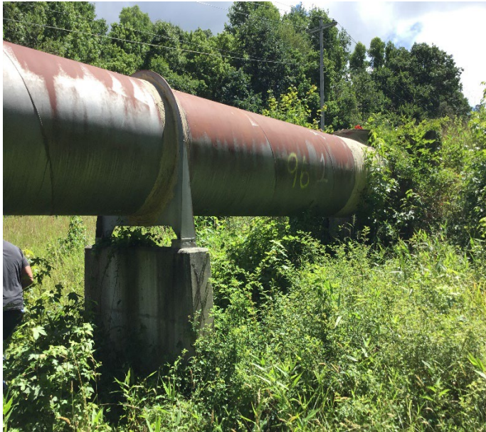
Picture of an existing saddle along the Richland Creek Outfall
