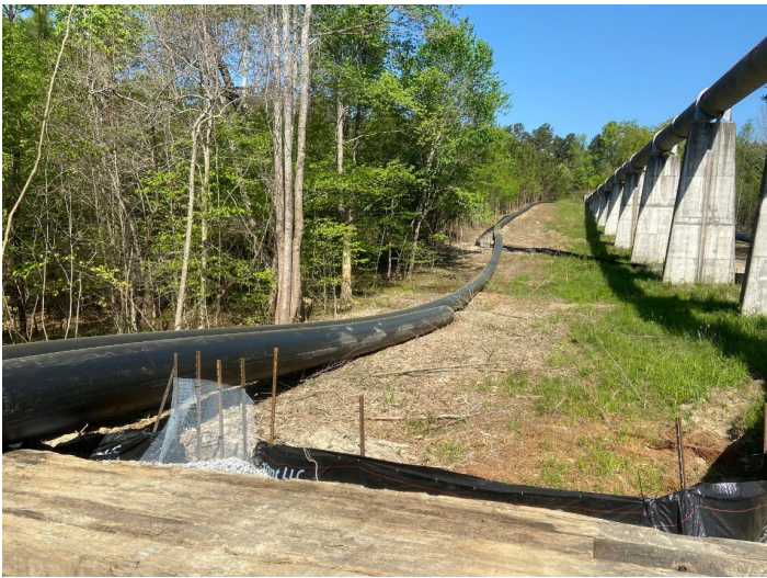
The leachate pumping system will discharge into the 24" Richland Creek bypass (black pipes on ground)
