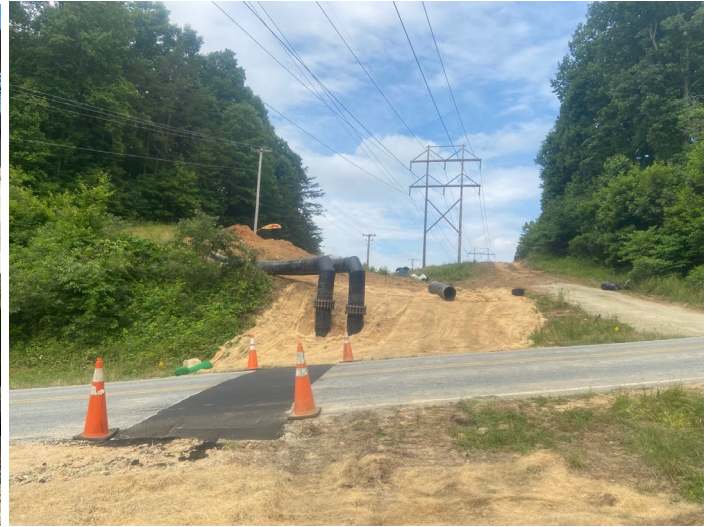
The leachate pumping system will discharge into the 24" Richland Creek bypass (black pipes on ground)
