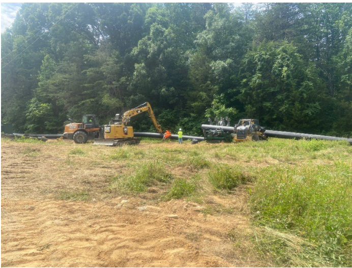
Construction crews are currently installing the 24" Richland Creek bypass piping. The leachate pumps will be similar to the orange pumps as shown above.
