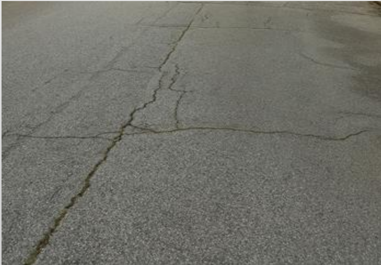
Reflective Cracking (Woodbrook Drive)
