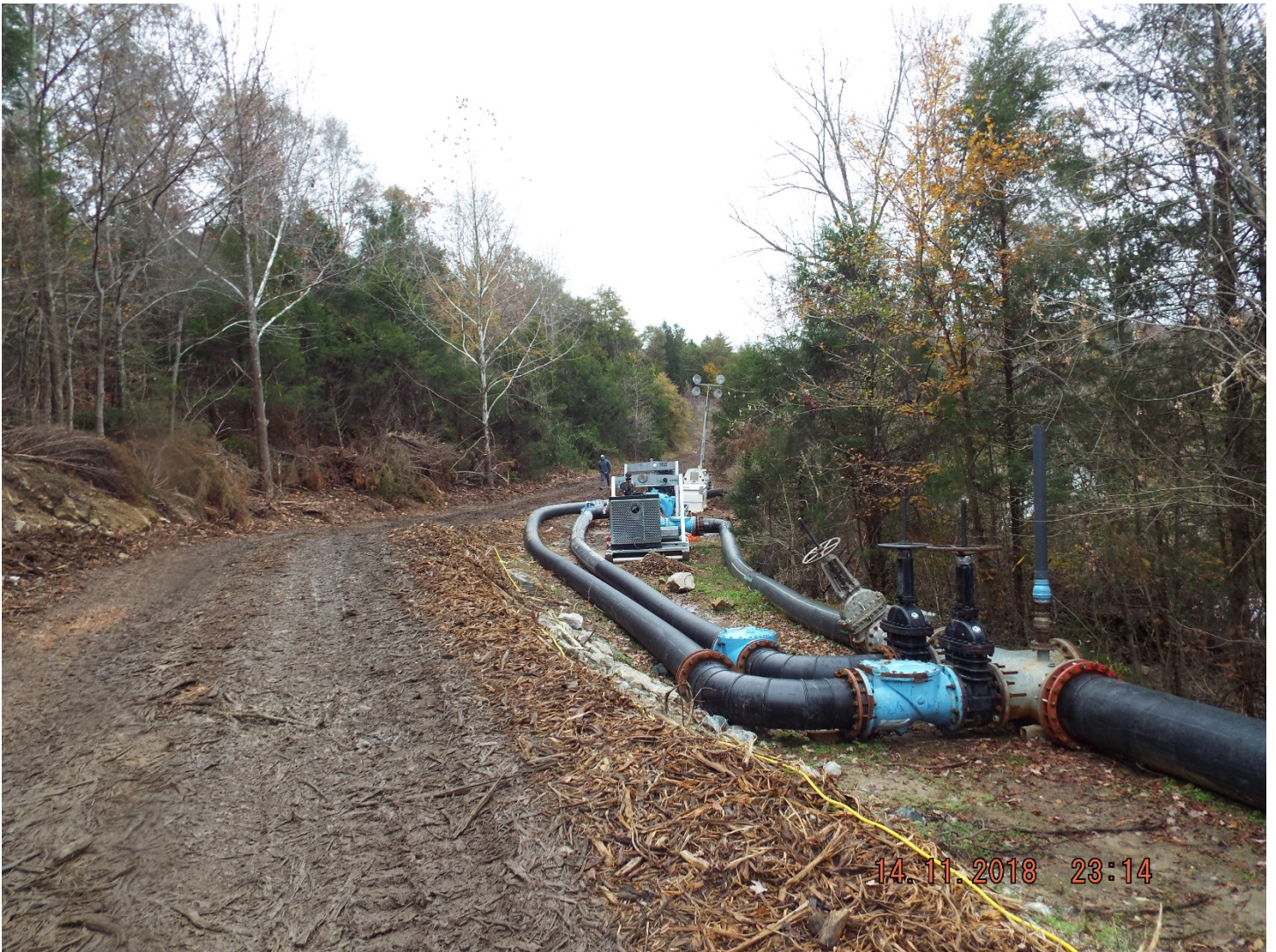
Picture of Riverdale Pump Station Bypass
