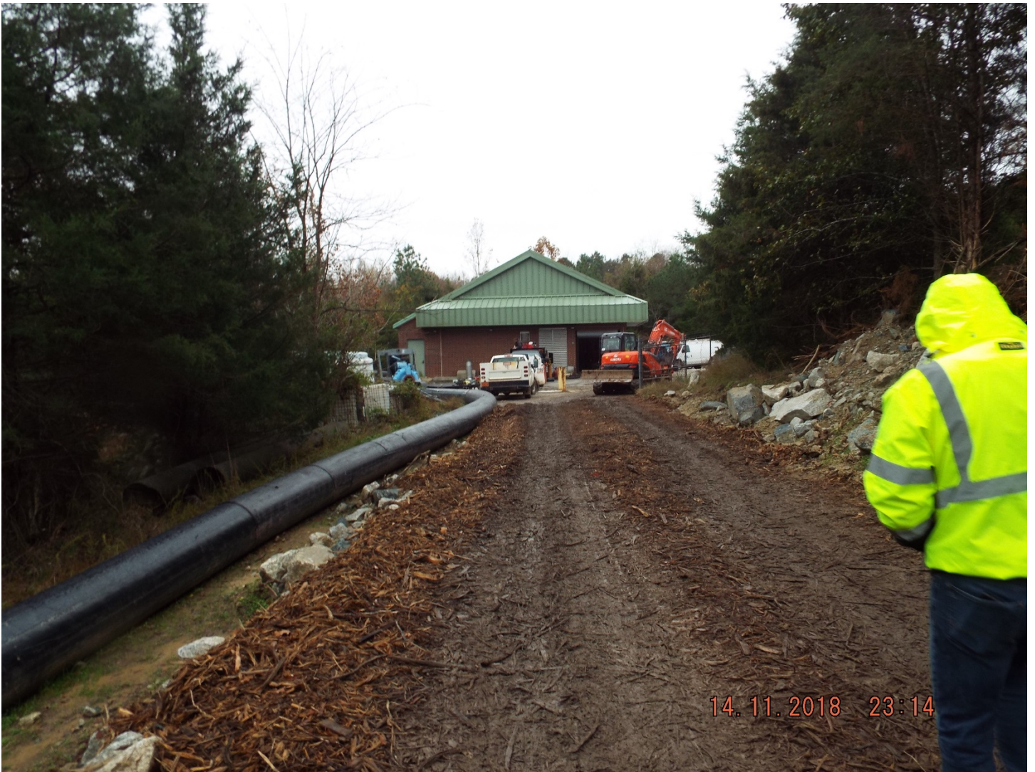
Picture of Riverdale Pump Station Bypass
