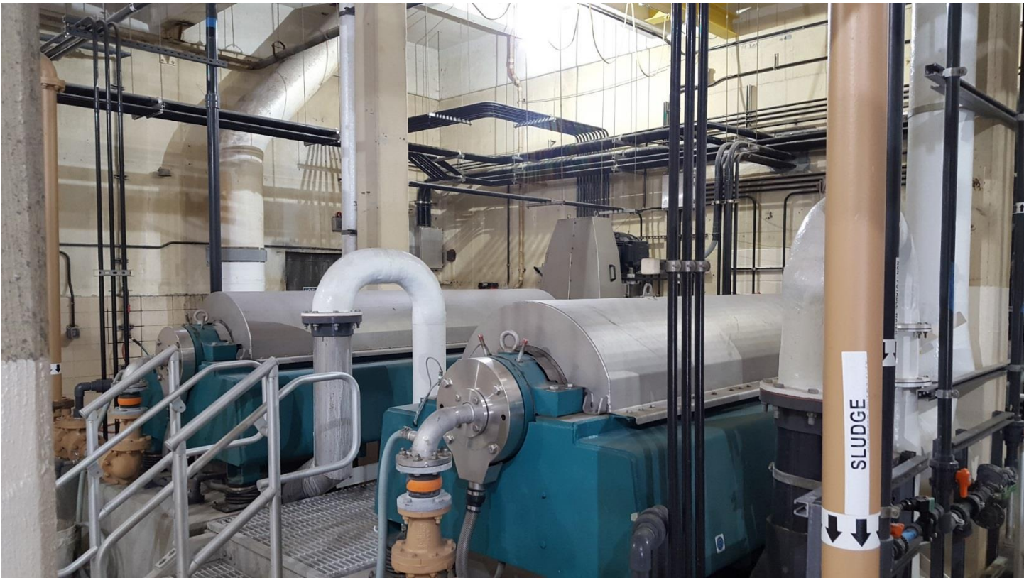
Eastside WWTP Centrifuges 1 and 2
