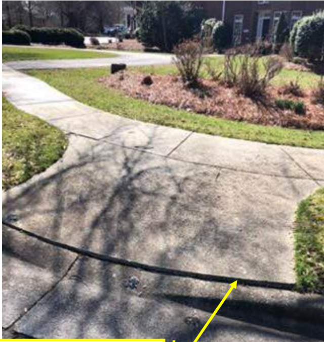
BOTTOM HC RAMP MOST SEVERE TRIP AND FALL HAZARD REPAIRABLE USING PRECISION CONCRETE CUTTING
