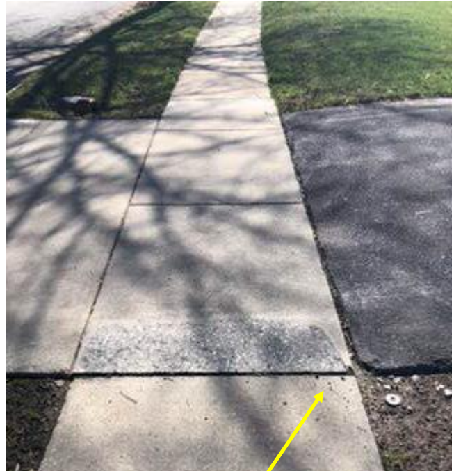
PARTIALLY REPAIRED WITH GRINDING MACHINE SEVERE TRIP AND FALL HAZARD REPAIRABLE USING PRECISION CONCRETE CUTTING
