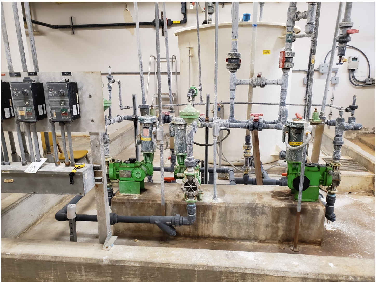
Picture of Existing Alum Feed System
