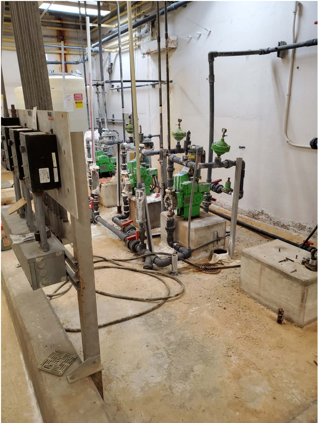
Picture of Existing Caustic Feed System
