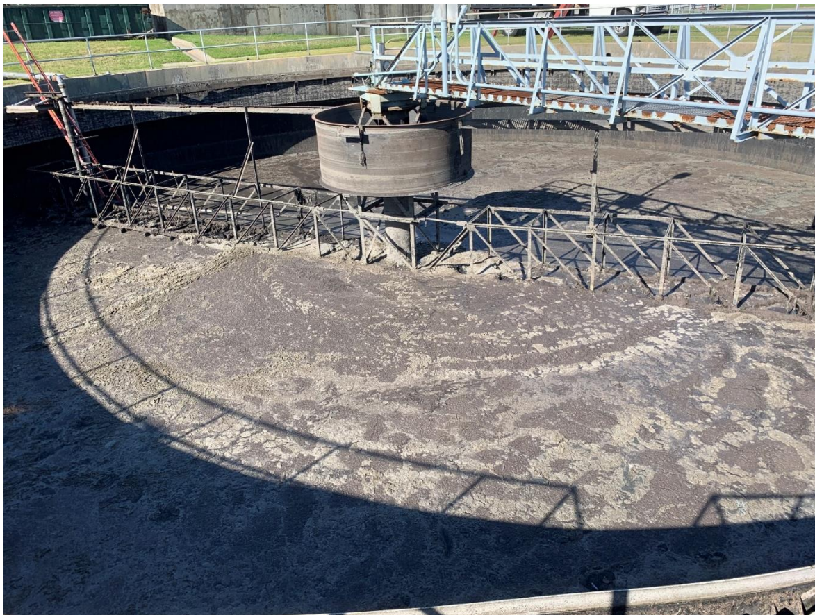
Primary Clarifier #1- Grit/solids accumulated above the bottom of the rake arm.
