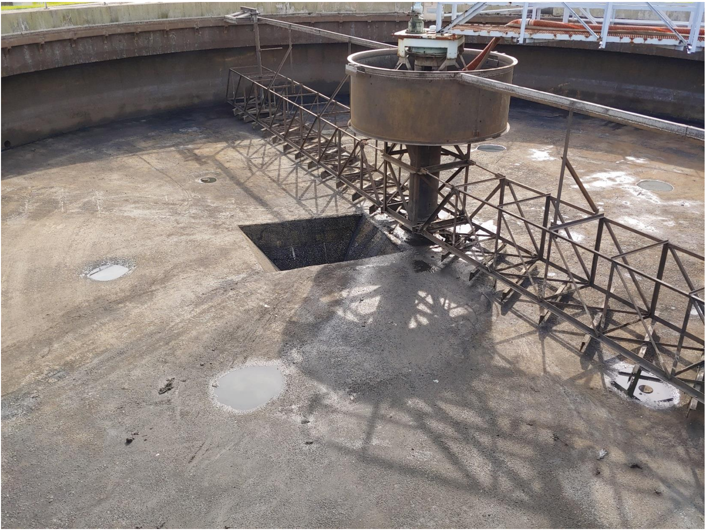
Picture of a primary clarifier after being cleaned out.
