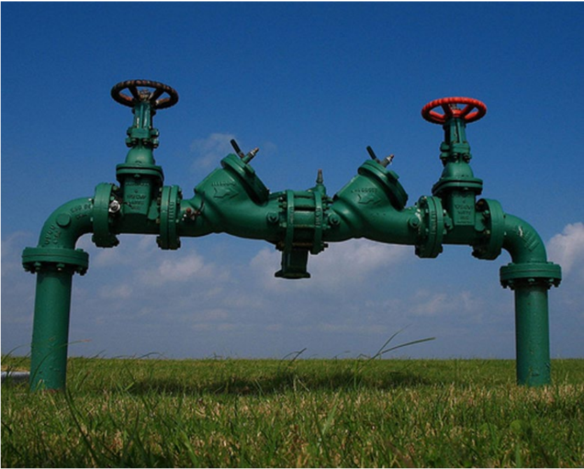
Example of a larger backflow device (commercial)
