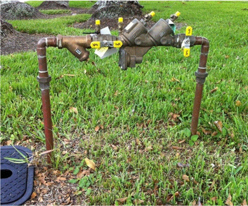
Example of an irrigation backflow device (residential)
