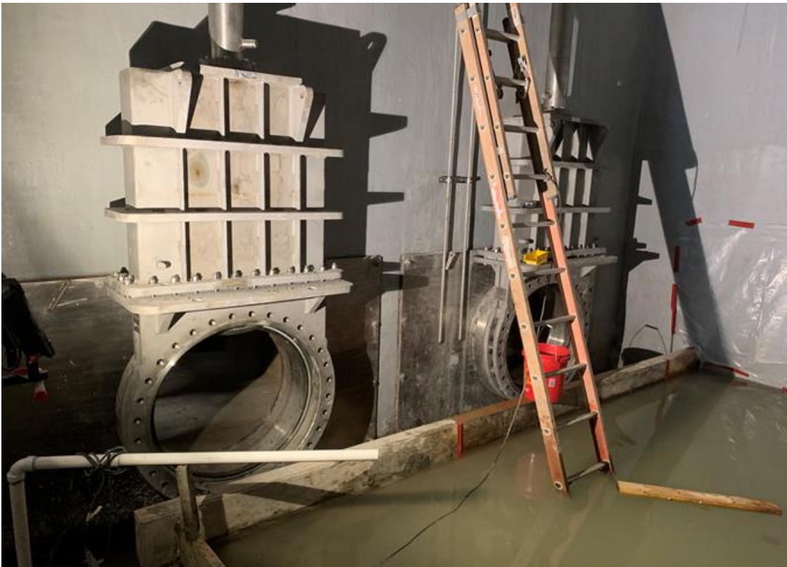
Knife gate valves installed in the wet well
