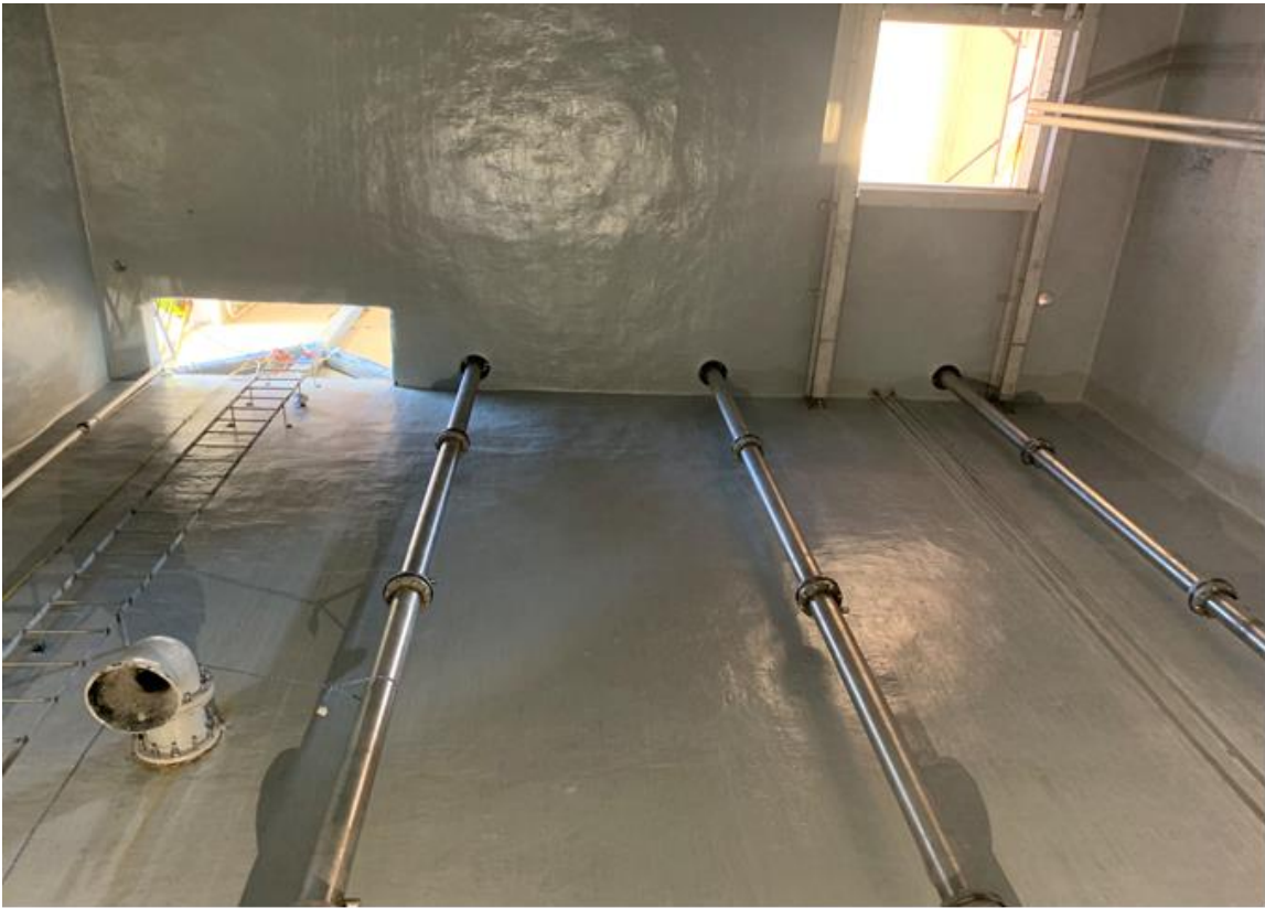
New wet well coating, ladder, and shafts for the knife valves
