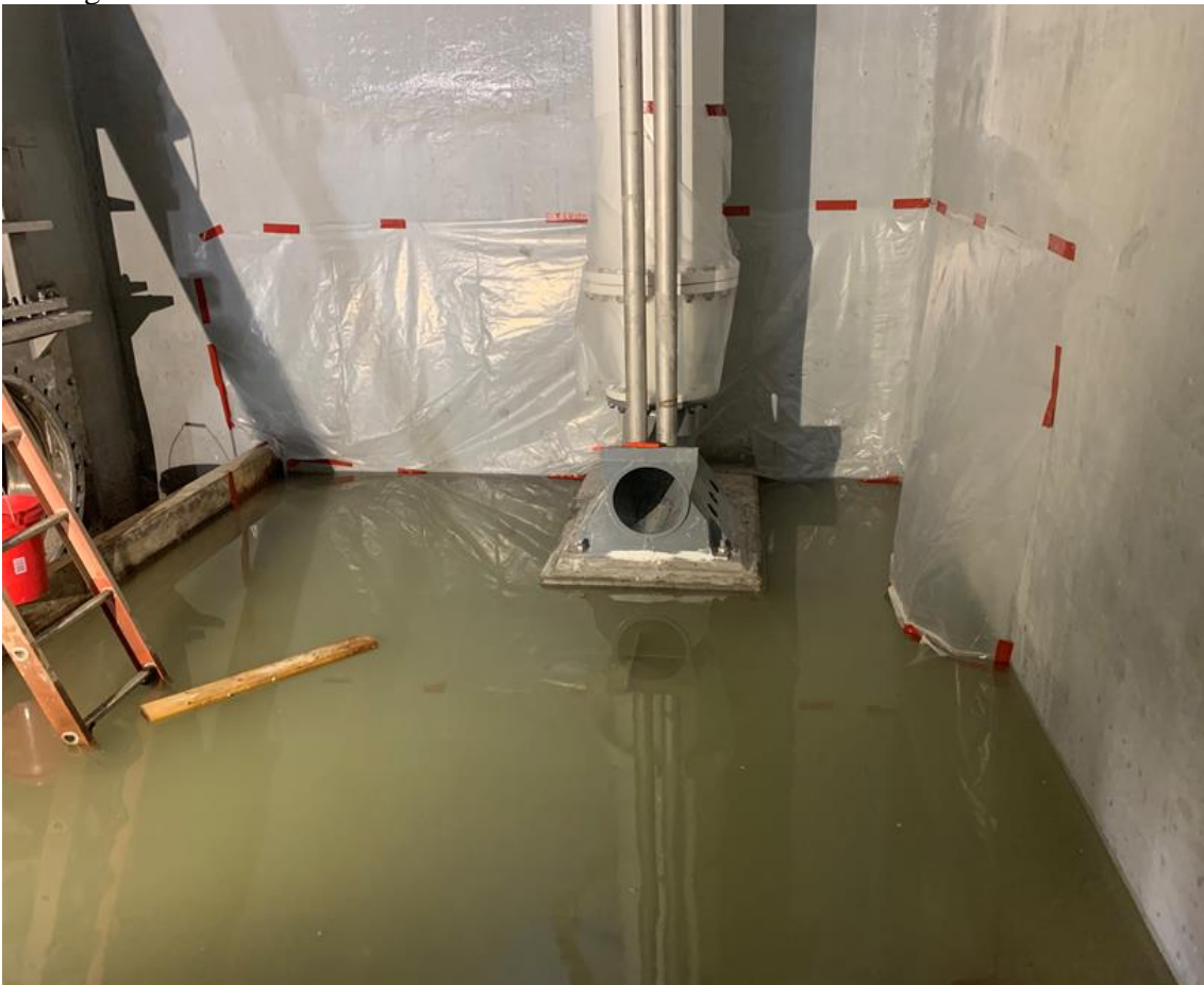
Connection for the new submersible pump
