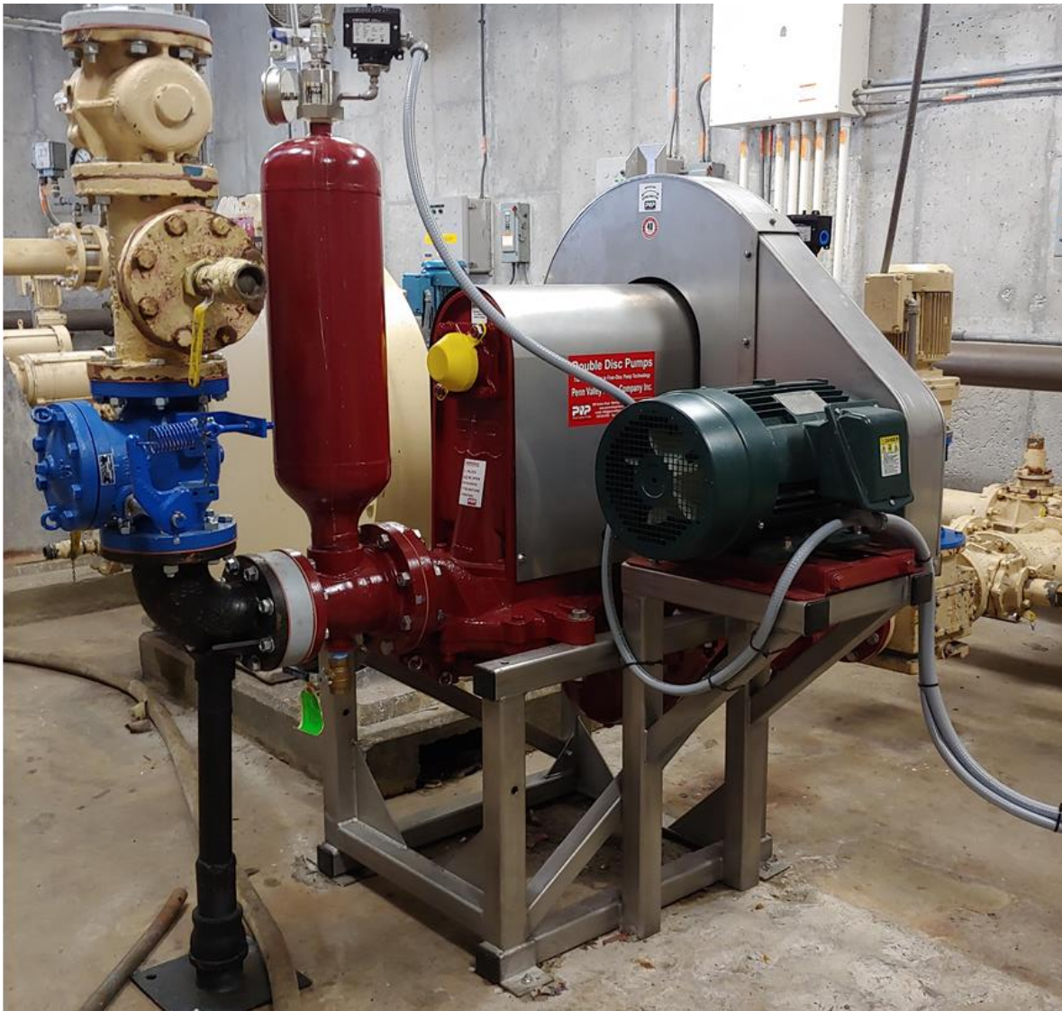
6" Penn Valley Double Disc Pump- Installed for trial testing in the Primary Clarifier Building
