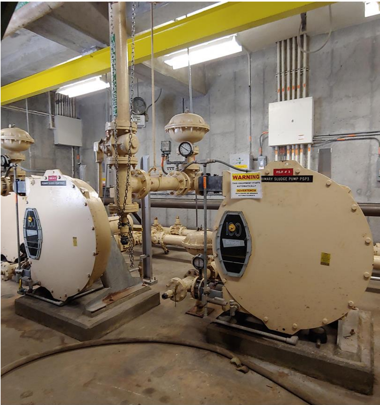
Existing Primary Sludge Peristaltic Pumps
