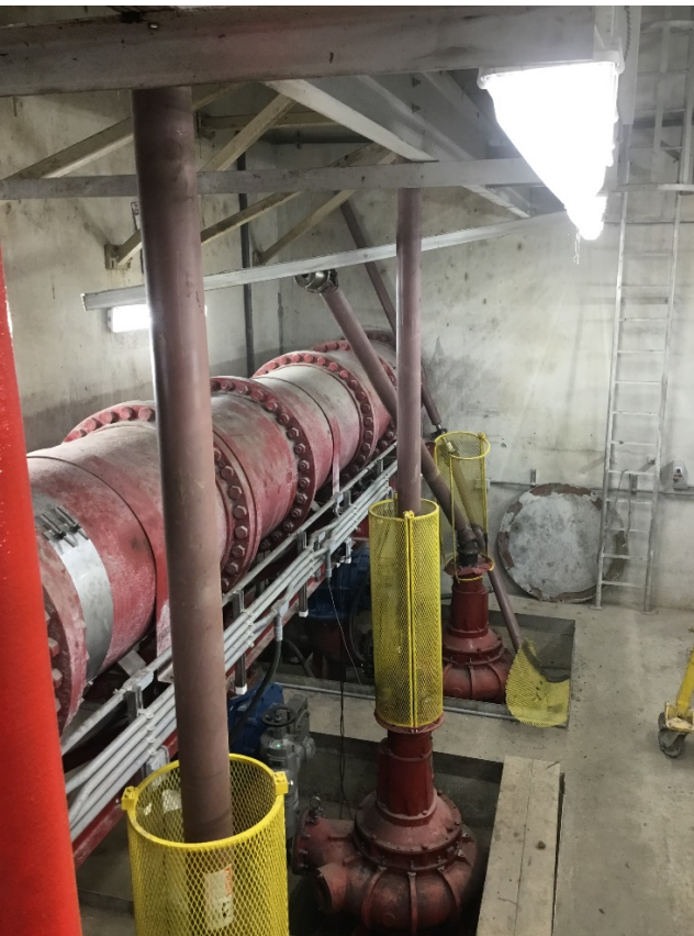
10 MGD Wemco-Hidrostal Pumps and Drive Shafts
