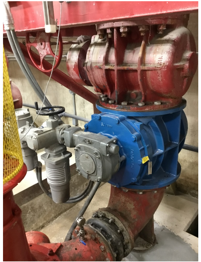
Newly Replaced 18" Plug Valve
