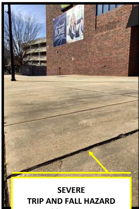
SEVERE TRIP AND FALL HAZARD Repairable using Precision Concrete Cutting Process
