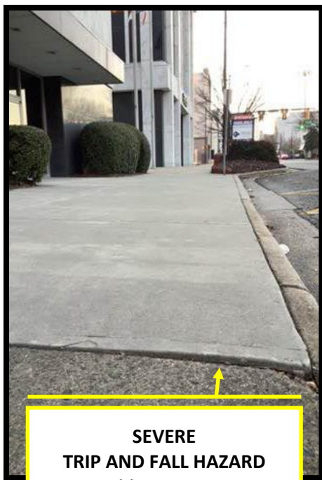
SEVERE TRIP AND FALL HAZARD Repairable using Precision Concrete Cutting Process
