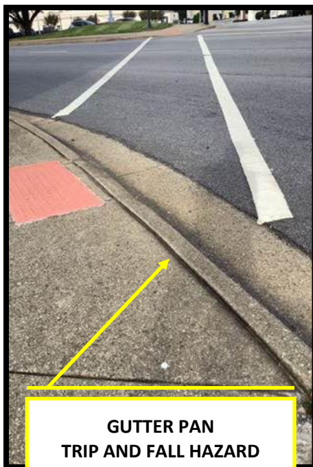
C2B TRIP AND FALL HAZARD Repairable using Precision Concrete Cutting Process
