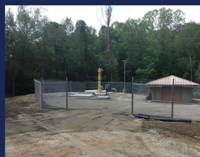
Construction of a new lift station with a peak capacity of 4.2 MGD and approximately 16,577 LF of 18-inch force main.
